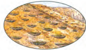
4 curved walls built from stones. Soil washed downhill collects behind them to form mini-terraces
